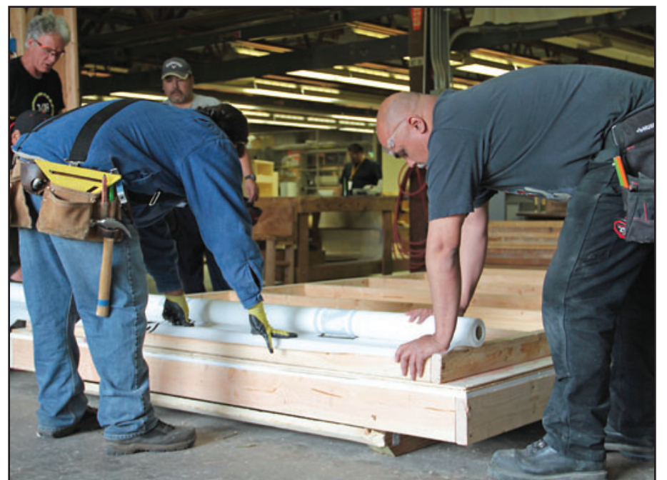
The approximately 8' x 12' structures each take five to ten days to complete and will be delivered to Nickelsville on June 9.
