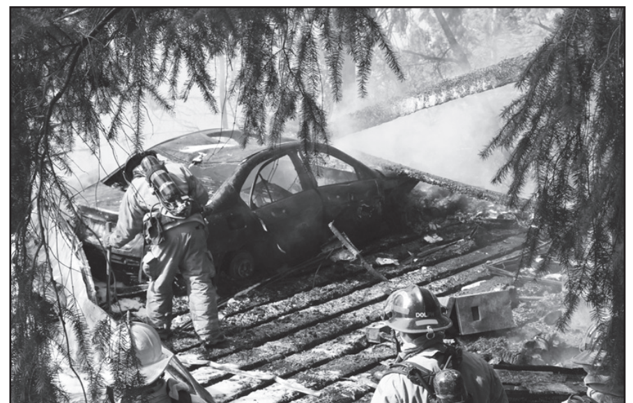
Firemen test the burnt out garage floor to reach the remains of the vehicle.
