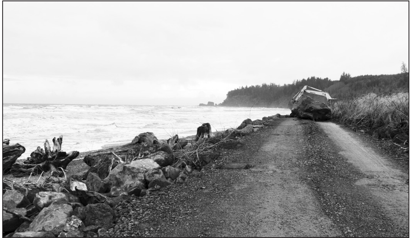
An access ramp was built to allow equipment onto the seawall for removal of capstones, and placement of a filter blanket armor rock.
