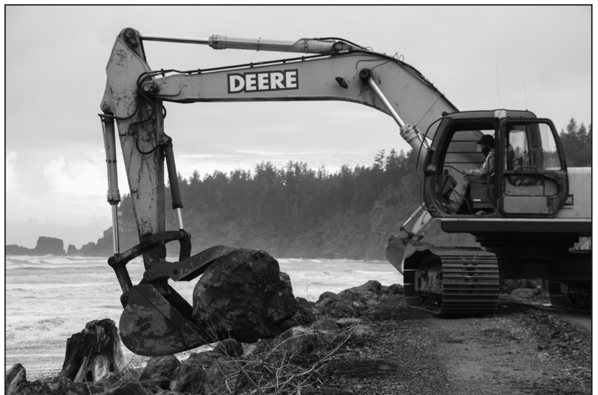
Placement of armor rock was conducted on Saturday, March 29, which will help decrease the vulnerability to wave action to the slope.
