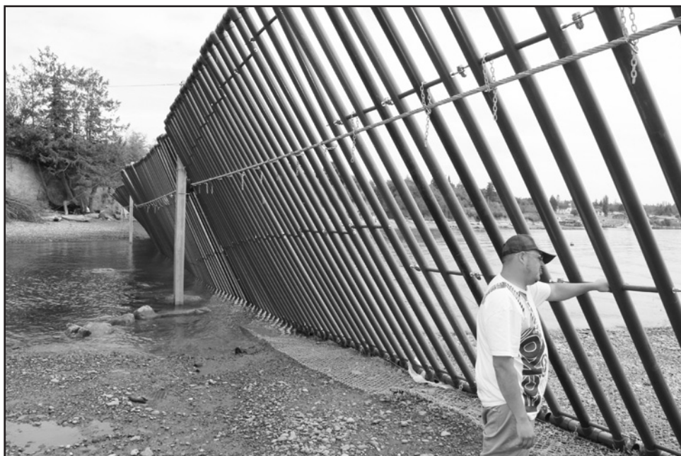
Jesse Rude, hatchery assistant manager, gazes through the fence that prevents sea lions from going up stream, while allowing salmon to pass through.
