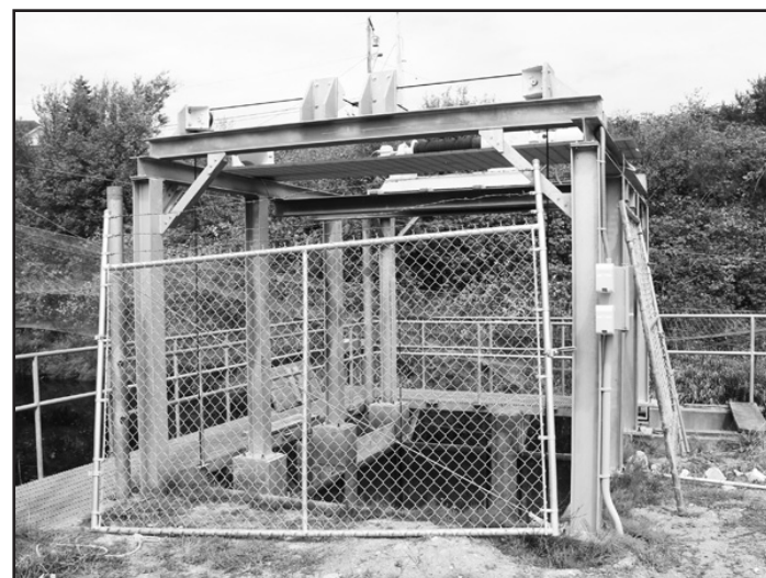
The redent addition of a mechanized holding pen and fish lift allows the salmon to be pulled out and processed more quickly than pitching fish by hand
